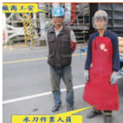
▶ Check water jet operator devices on site
