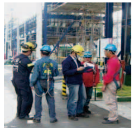
▶ Ask construction personnel for JSA questions
