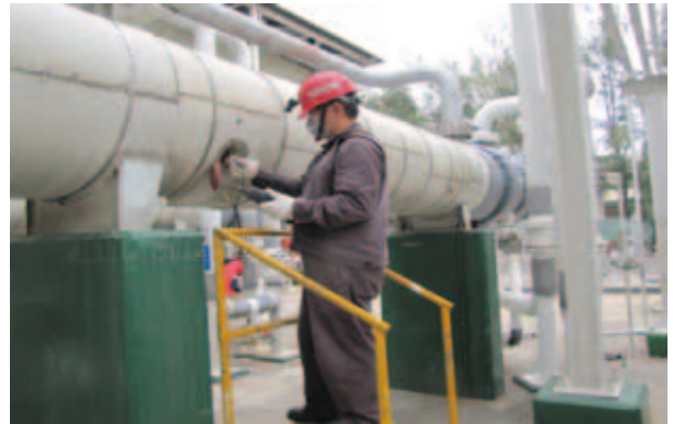
▶ Ergonomic hazard improvement case (after)
