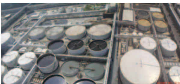
▶ Wastewater Treatment Plant (Before improvement)
