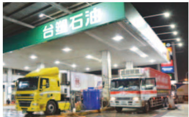
▶ To respond to energy-saving policies of the government, we have installed LED projecting lights and pendant lights to keep stations trim and bright.
